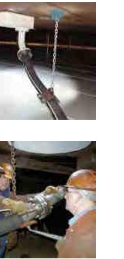
CTS tank drain hoses are a proven solution for the challenging draining of rain water on external floating roofs. The major advantage of these hoses is its simplicity in design. It has a limited amount of connections and therefore high reliability. To avoid floating the CTS drain hose includes a lead ballast cable and suspension system. All hoses are supplied electrically continuous to prevent buildup of static electricity.
