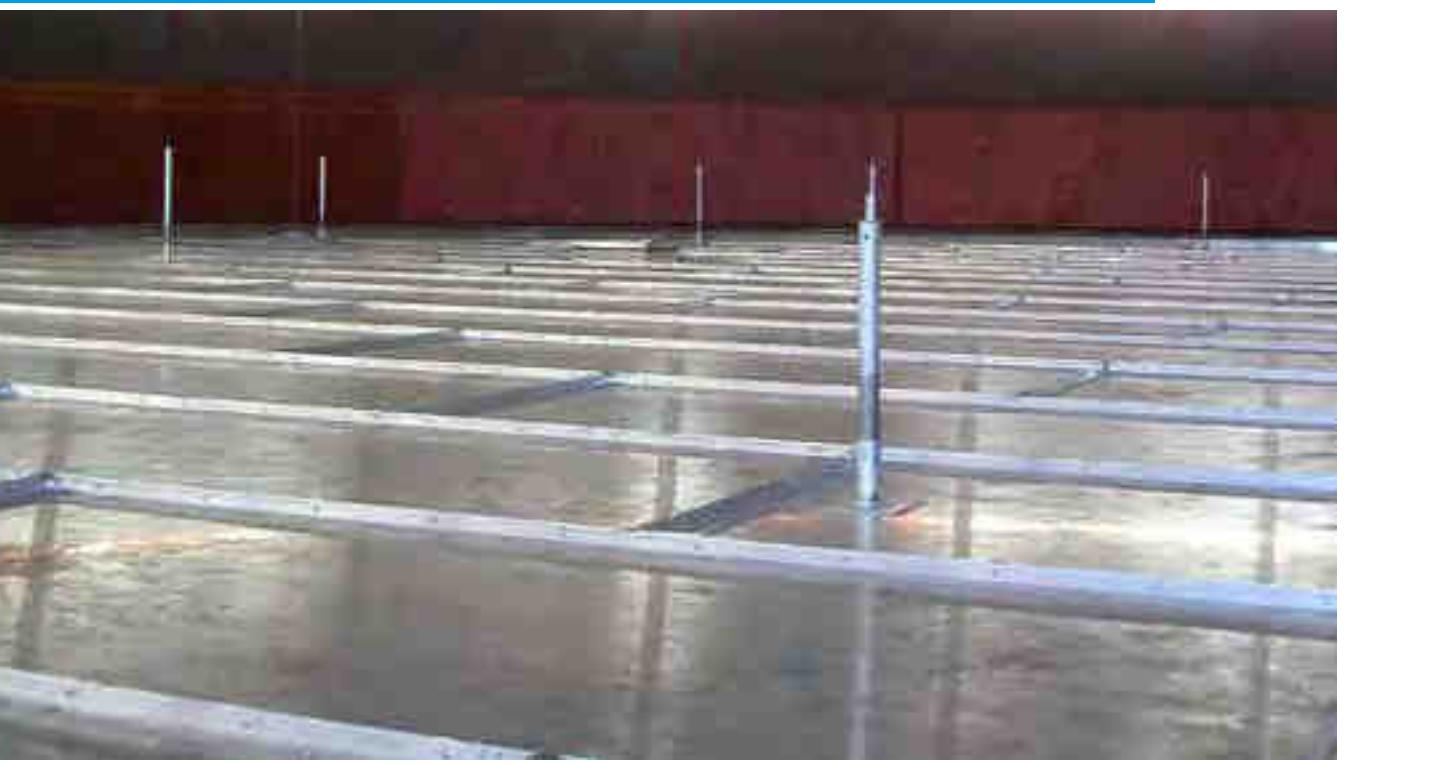
The most efficient solution for reduction of VOC (Volatile Organic Compound) emission on storage tanks is the direct contact IFR. Full contact Internal floating roofs (IFR's) eliminate these emissions at the source.
