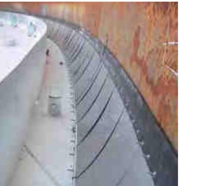
The CTS40 is a double rim mounted compression plate tank seal (primary and secondary seal). Its design is based on compression plates pushing a rubber tip against the tank shell. Behind the compression plates, fully shielded from weather exposure a vapour barrier fabric ensures the vapour tightness of the seal.
