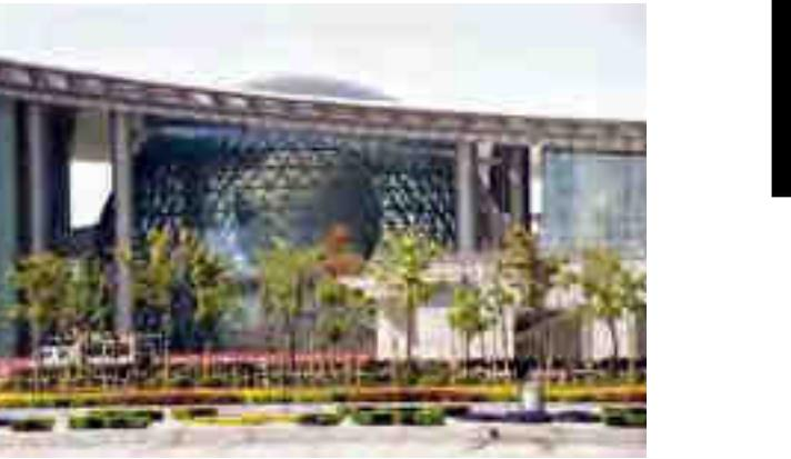
The aluminium dome is a unique triangulated space truss skinned with aluminium panels secured by a patented batten closure system. With an ability to offer clear spans from 10 to more than 300 meter aluminium domes are specified for large covers area's such as churches, sports arenas, exhibition centres. Aluminium domes are as beautiful as they are efficient and durable. Aluminium integrated structural frames are permanent and lightweight. Optional panel systems offer eye-dazzling options.
