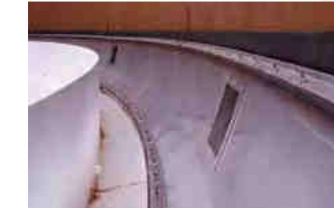
The CTS 20 is the most common design for secondary tank seals. It consists of compression plates pushing a rubber tip against the tank shell. Behind the compression plates, fully shielded from weather exposure, the vapour barrier fabric ensures the vapour tightness of the seal.
