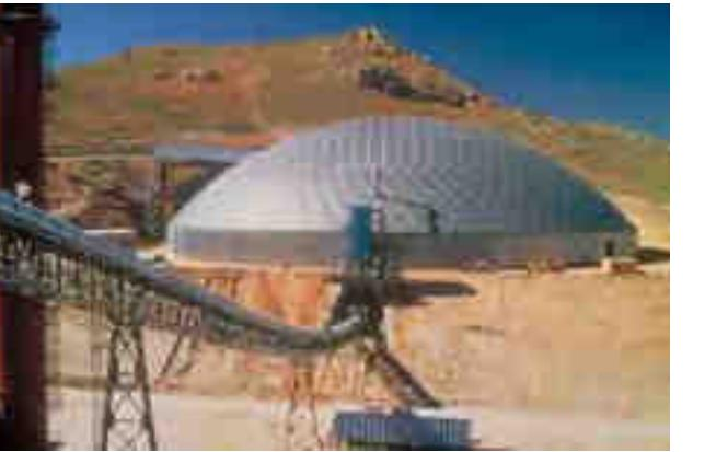
CTS aluminium domes are the ideal solution for dealing with challenging environmental enclosure. Whether it is keeping the elements out or getting the largest amount of bulk in the smallest amount of space, an aluminium dome has proven to be the optimal solution. Domes offer the ideal span-to-rise ratio in standard and custom designed configurations for any clearance requirement.
