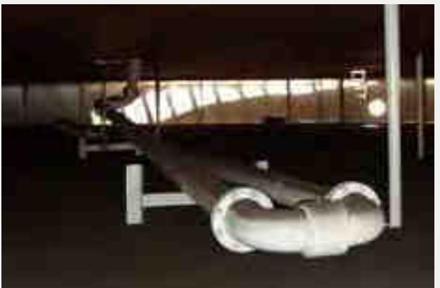
Tanks drain systems can only be replaced when the tank is out of service, therefore the consequence of a malfunctioning tank drain is significant. To ensure long service life CTS has developed a tank drain pipe solution with high quality swivels. The CTS drain pipe system is a complete system, including the connections, swivels and the piping required. Please refer to the swivels leaflet for more information on our swivels.
