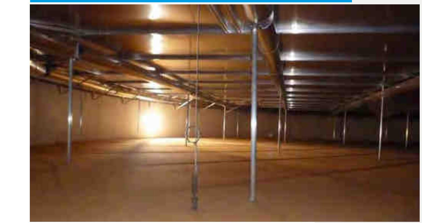
Pontoon type internal floating roofs (IFR) eliminate VOC emissions by saturating vapour and preventing new vapour to form. These skin and pontoon IFR are designed as light weight floating structure sealed with a closed skin. This design will reduce emission with more than 98%.
