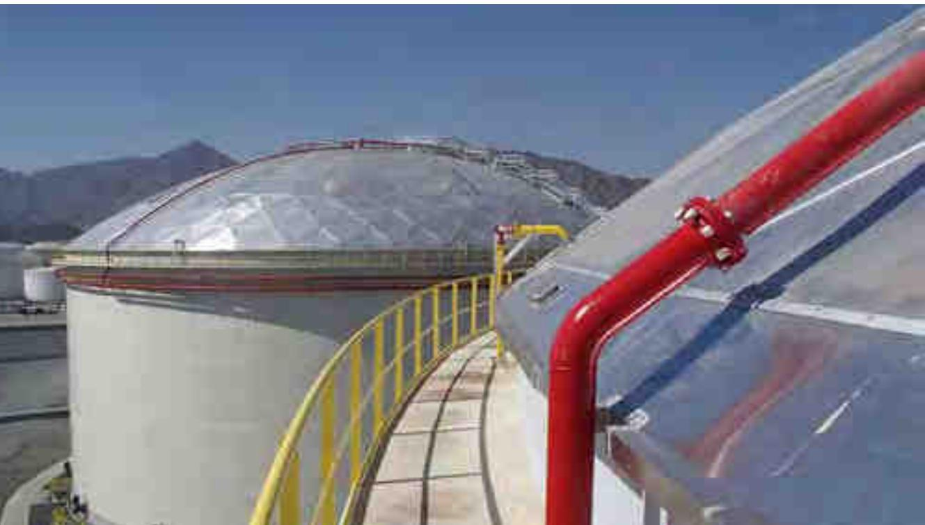
*The lightweight economical covering solution is ideal for covering steel external floating roofs, as cover for new tanks or even for replacement of the more traditional steel roofs on storage tanks. CTS offers a full solution from engineering to supply and installation, which is the only way to truly get all benefits domes have to offer. With over 1,500 domes supplied worldwide CTS is the leader in engineering supply and installation of these state of the art covering solutions.*
