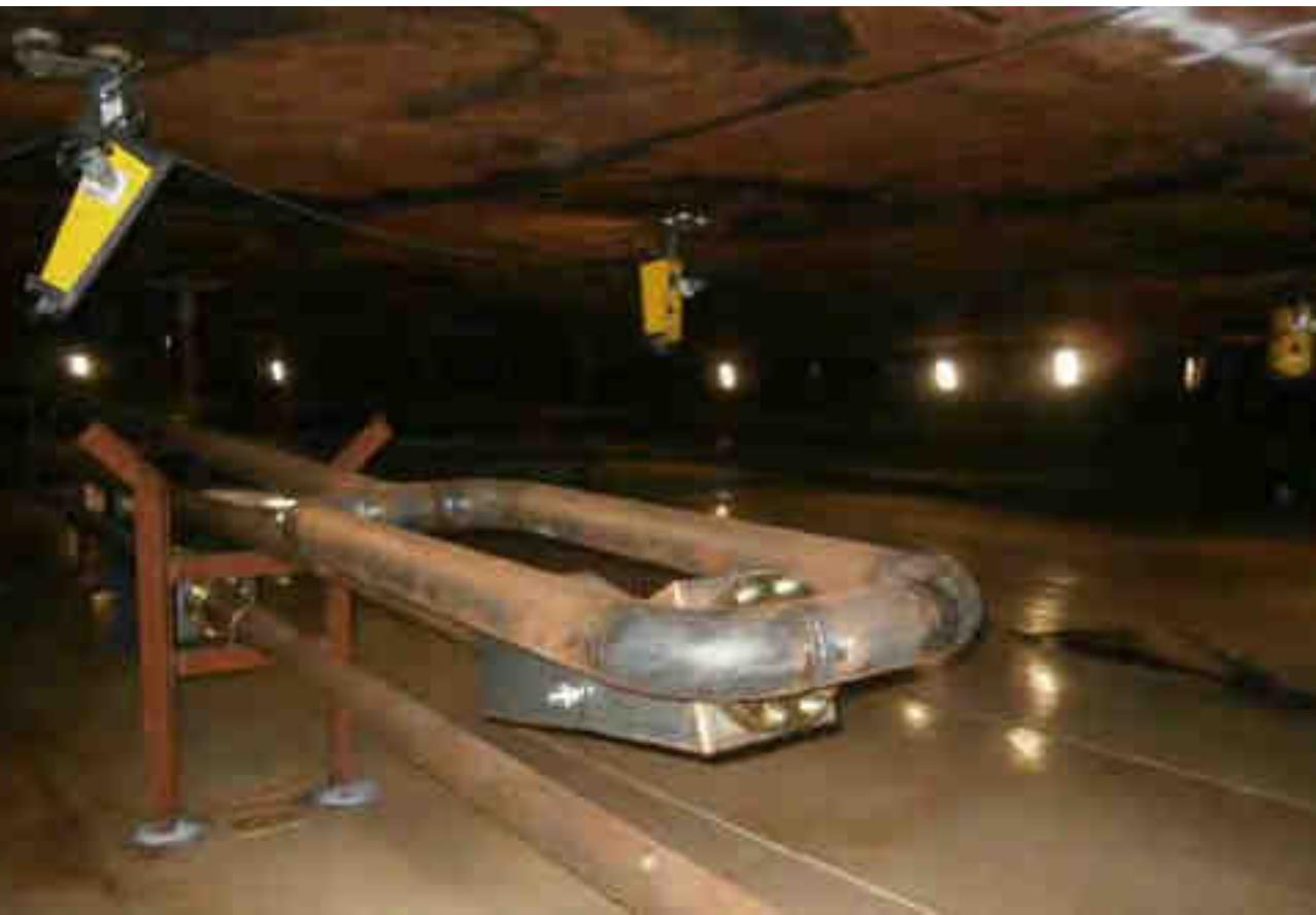
The drain master consists of a reinforced composite hose fitted in a metallic pivoting joint. This is an ideal long-lasting flexible pipe connection for this application.
