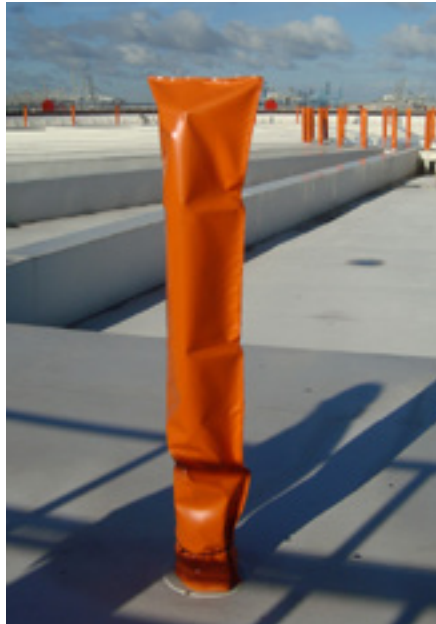
Leg sock on tank in service, PU (Polyurethane) fabric.
