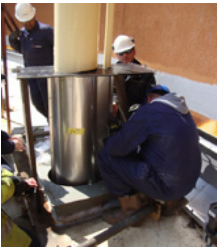
Gauge pole sleeve during installation.
