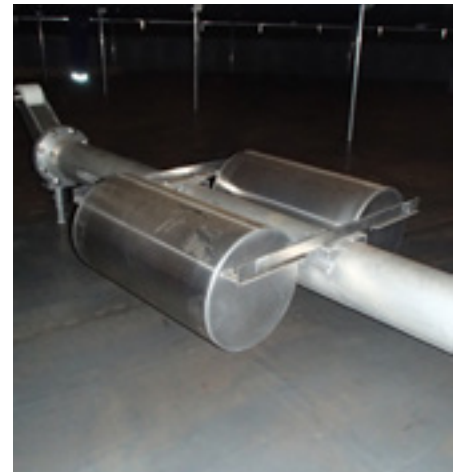
Floating suction line under internal floating roof.
