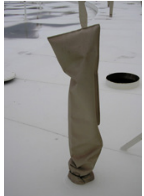
Leg sock on tank in service, PTFE (Teflon) fabric.
