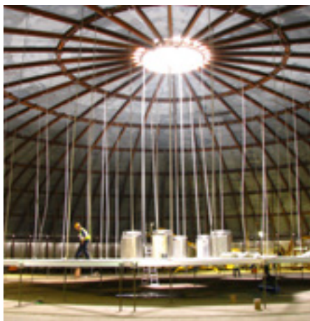
Completed Deck Prior to Dome Airlift.
