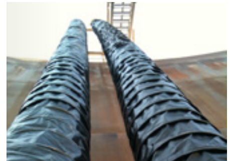
Gauge pole cover, view from floating roof.
