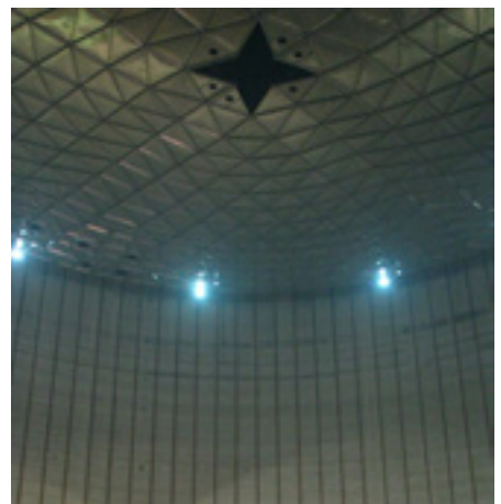
Bottom Side Completed View.
