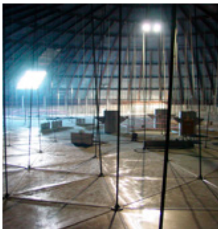
Topside Completed View.
