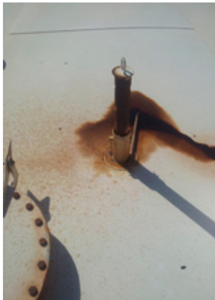
Leg seals will prevent product splashing out from leg sleeves.
