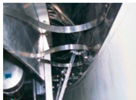
Liquid mounted shoe seal, bottom view.
